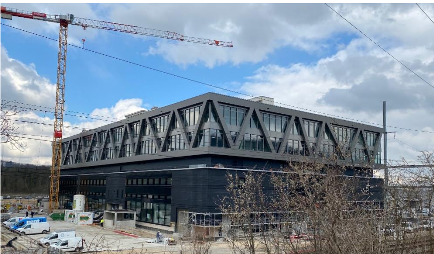
Caption: Construction progress at uptownBasel (source: uptownBasel)
